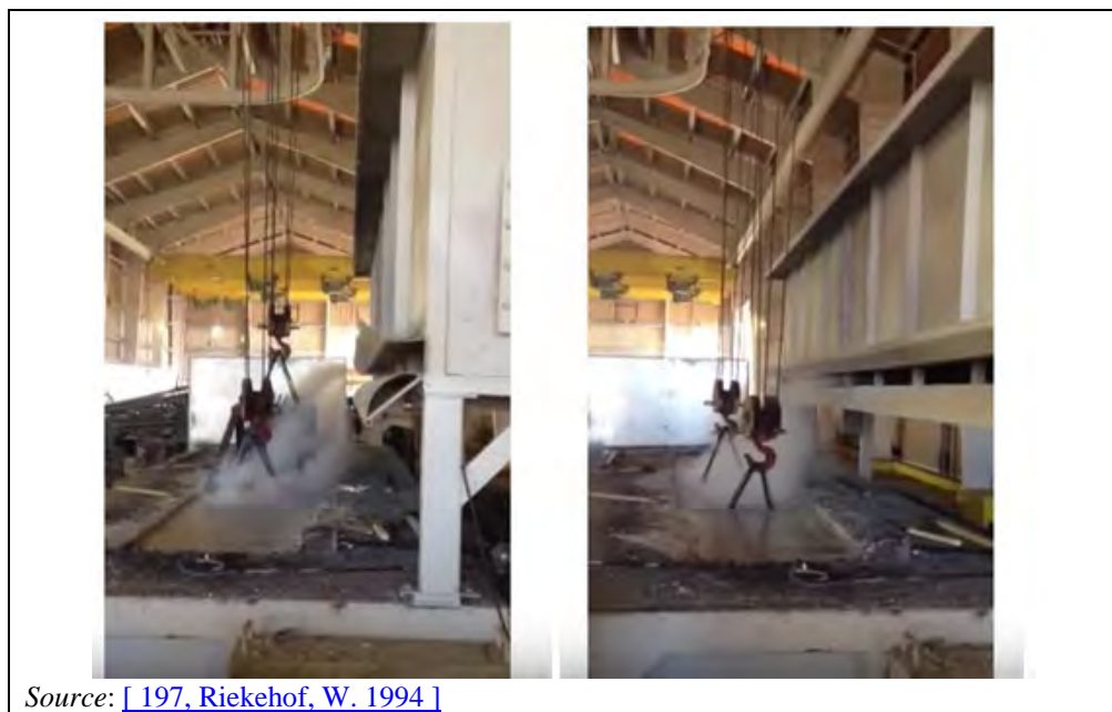
Figure 8.50: Lip extraction at a batch galvanising plant
