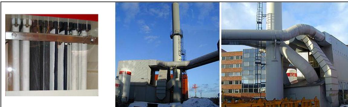
**Figure 4.10: Bag filter units; inside (l.) and outside (m., r.) views**
