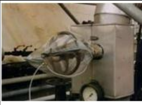
Figure 3.38: Bagging of a leaking valve
