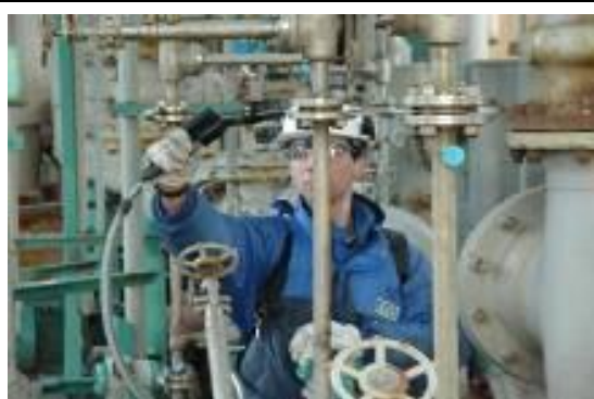
Figure 3.37: Leak concentration measurement
