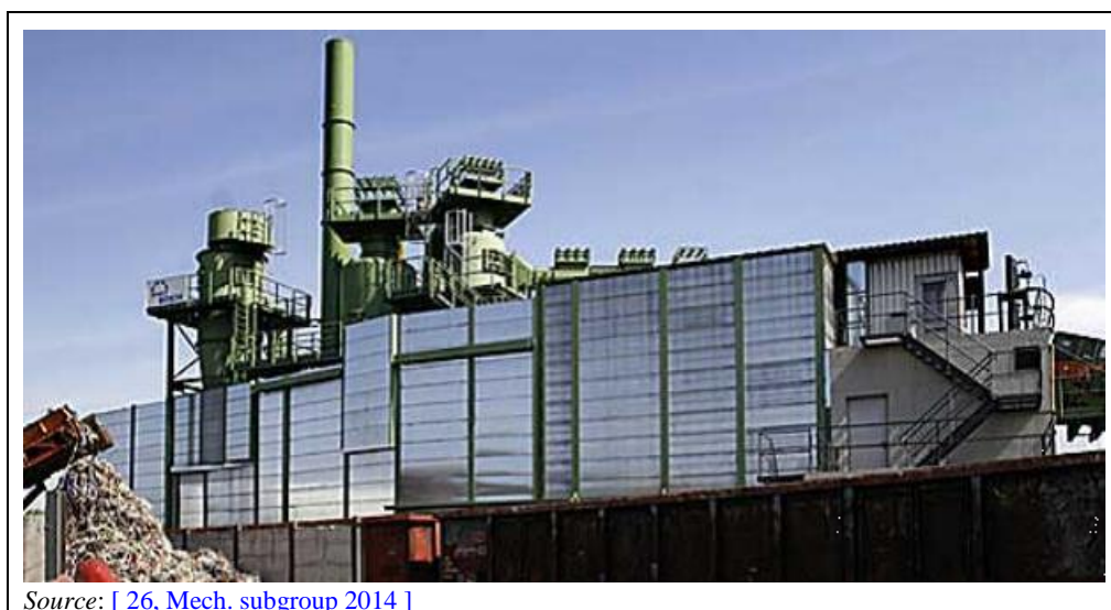
Figure 3.23: Protective screening at the Schrott-Bosch GmbH shredder, Germany
