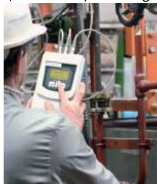
Figuur 3: controle via verificatiesoftware
