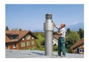
Figure 32: ESP fitted at the mouth of the chimney (Supplier information electrofilter, 2019)
