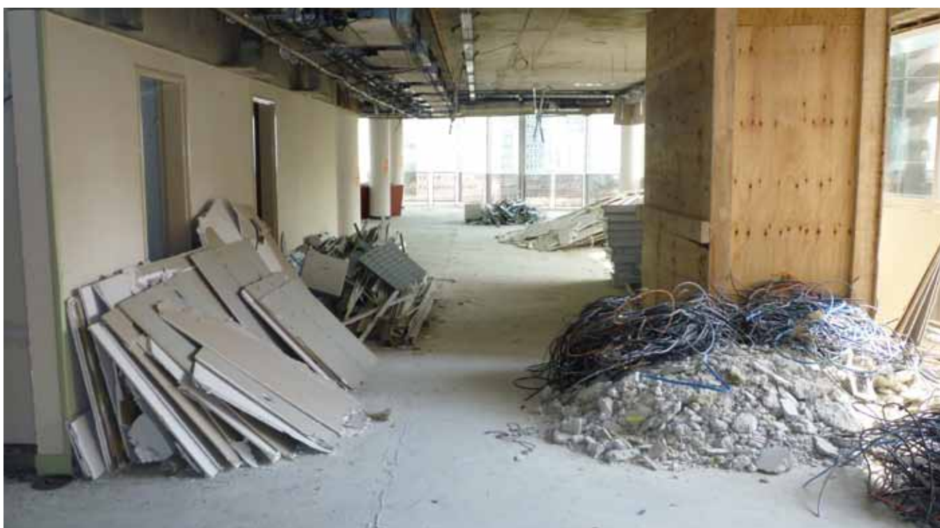
Gypsum sticks to other construction materials in demolition waste, making it difficult to valorise the material
