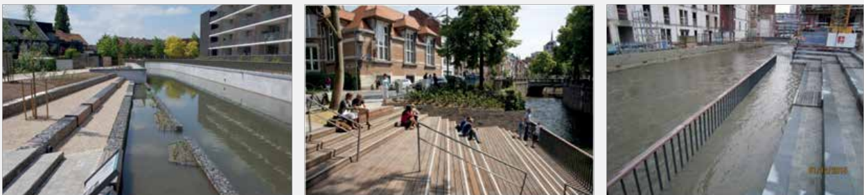
Photos: Terraces alongside the River Dyle in Leuven © Flanders Environment Agency
