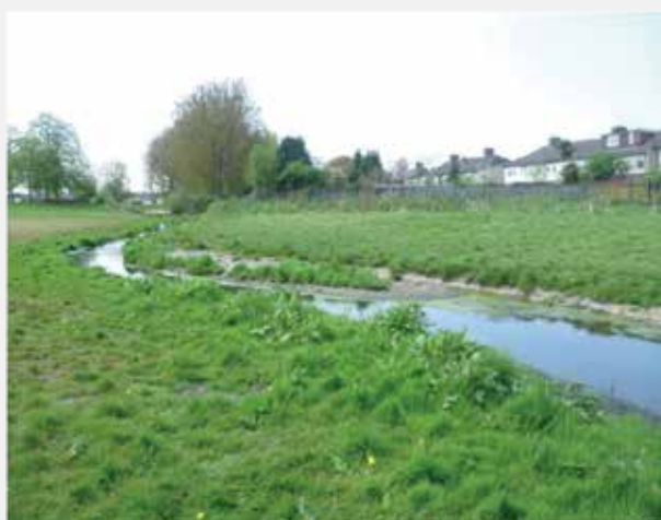
Photo: Reach on the River Mayesbrook over a year after restoration, showing rapid morphological recovery with vegetated banks and mid-channel bar formation © Environment Agency
