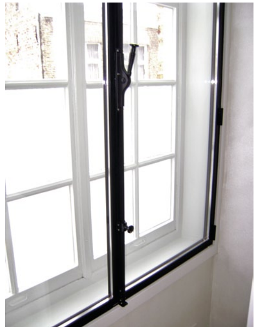
FIG. 77 Detail achterzetramen Veurne (foto Ines Deschepper)
