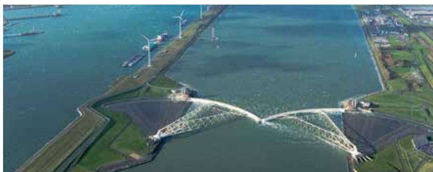
The Maeslantkering is a storm surge barrier in the Netherlands, which automatically closes when needed for protection.
