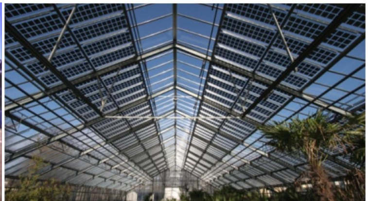
Figure 22 and Figure 23: PV on a sound barrier and in a horticultural application.
