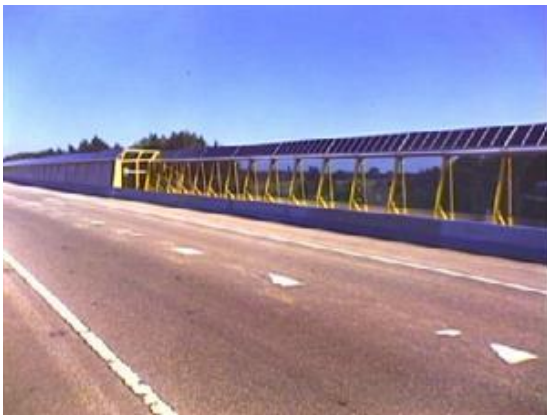
Figure 22 and Figure 23: PV on a sound barrier and in a horticultural application.
