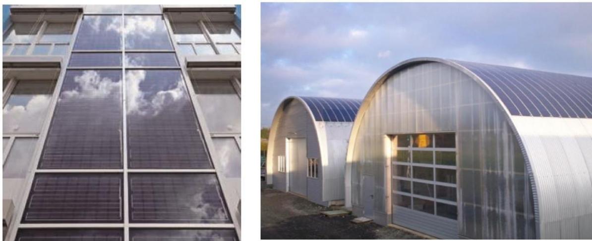
Figure 18 and Figure 19: A façade cladding PV solution and thin film PV solution on a curved roof.
