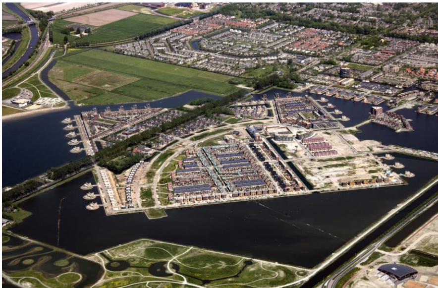
Figure 4: City of the Sun (photo taken during the construction phase, 2009), Municipality of Heerhugowaard.
