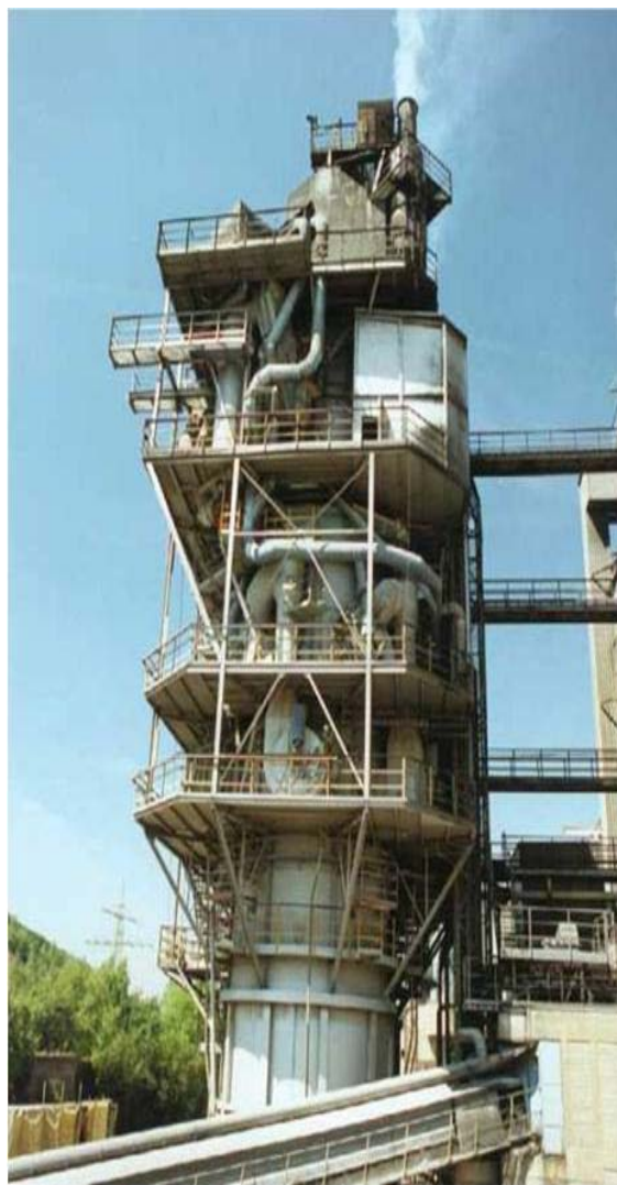
Figure 2.26: Example of an annular shaft kiln used in lime manufacture1
