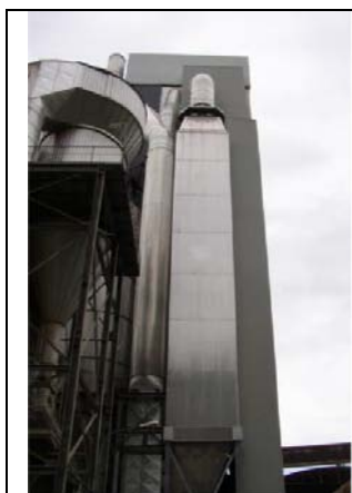
Figure 1.66: Example of an SCR installation Source: [140, Italy, 2007]
