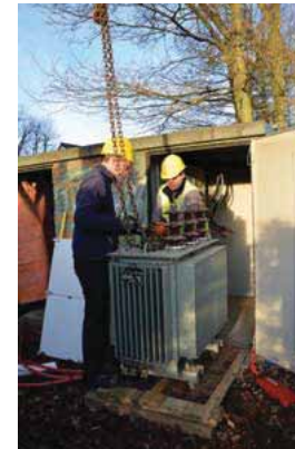
Figure 27: the transformer in Bret-Gelieren was replaced by a new transformer with oil temperature measurement equipment.
