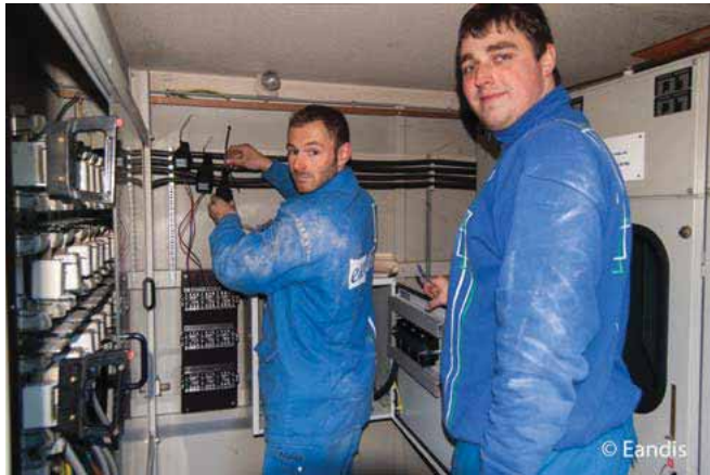
Figure 67: installation of measurement equipment at an Eandis transformer.
